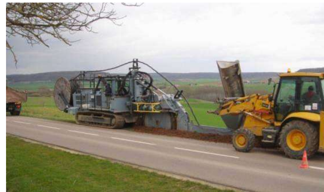
Figure 28 : Figure 29 : Trancheuse et raccordement
